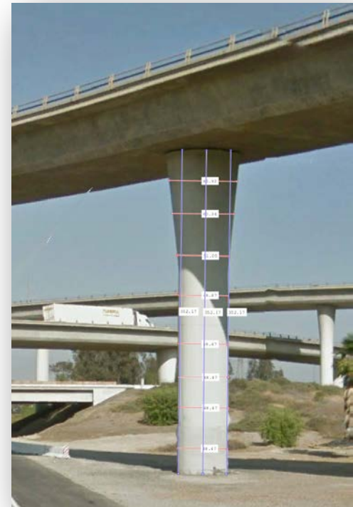
Determination of column dimensions
